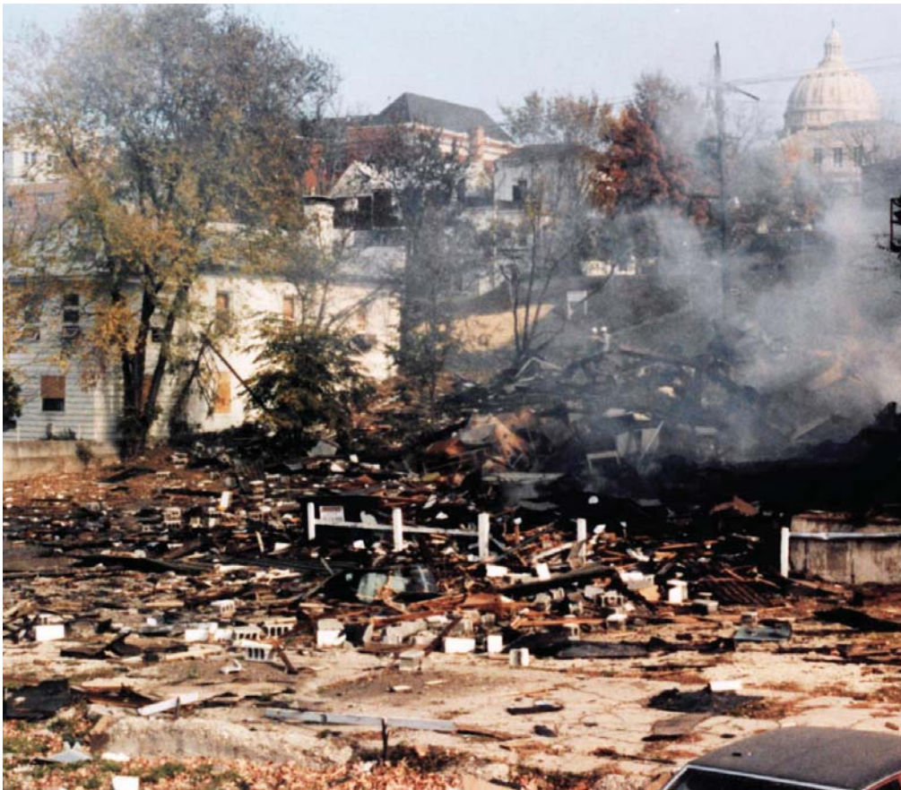
The remains of an office building explosion in Jefferson City in 1988.
